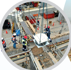
Over 1,100 base isolators were installed on the basement columns
